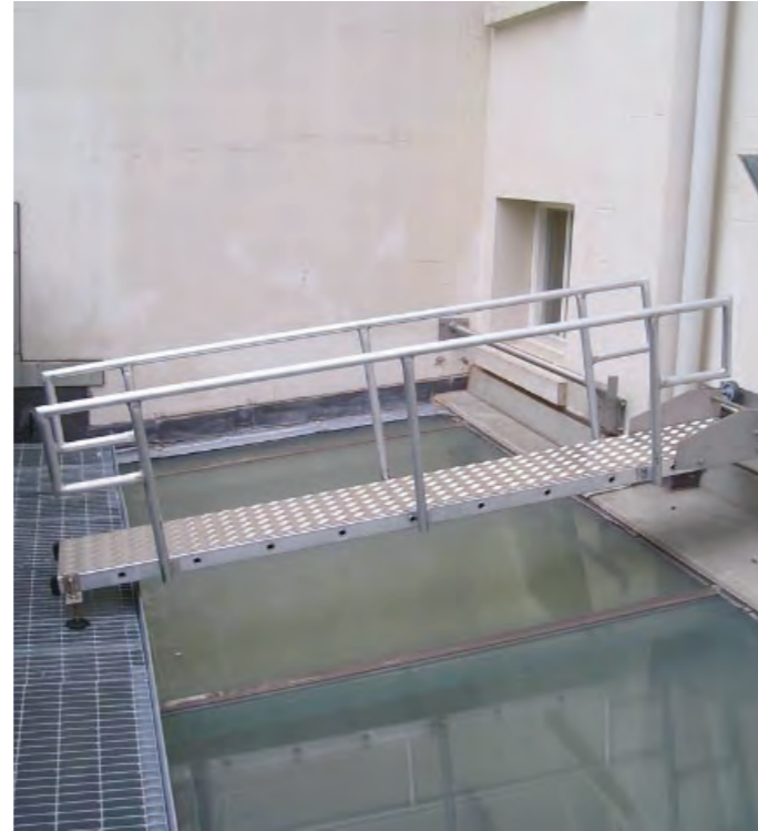
Fig 3. Greenwich University Purpose deigned alloy walkway on moving track over glass roof.
