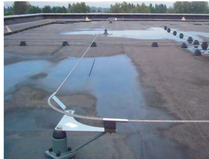
Flat concrete bitumen roof
