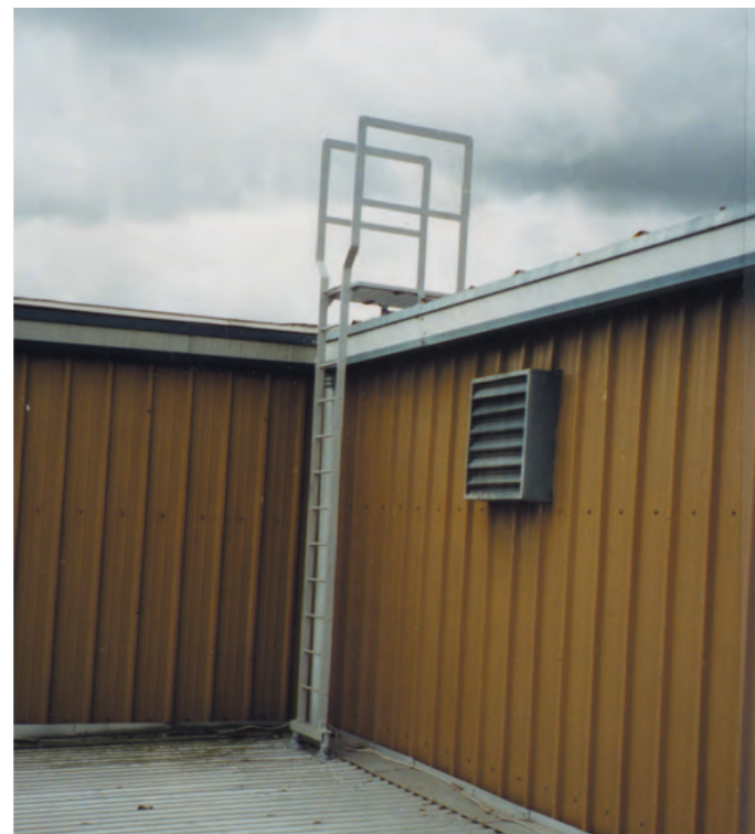
Fig 3. Industrial Warehouse Galvanised steel access ladder
