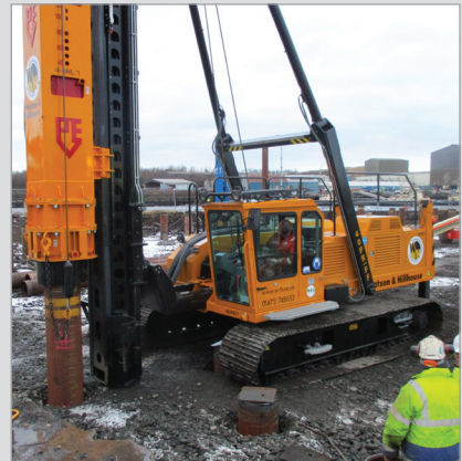
Piling and drilling rigs
