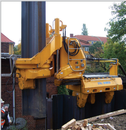
Kowan Still Worker noise and vibration free pile pressing machines
