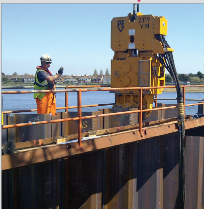
Crane suspended and excavator mounted vibratory hammers
