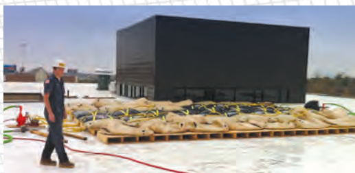
Roof load testing using Enclosed Water Load Test Bags.
