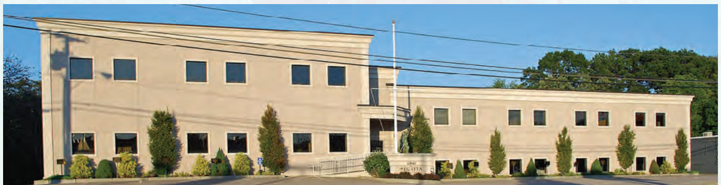
SUBSALVE USA corporate headquarters and state of the art manufacturing facility located in North Kingstown, Rhode Island, USA.
