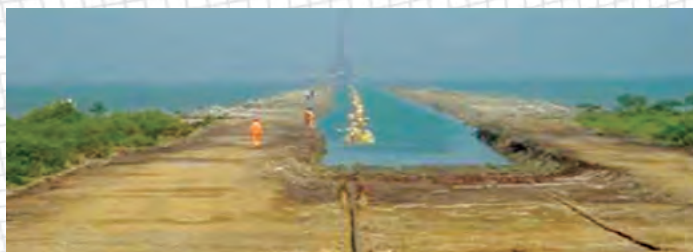
Installation of oil pipeline in the Middle East using Salvage Pontoons 6,000 lbs.
