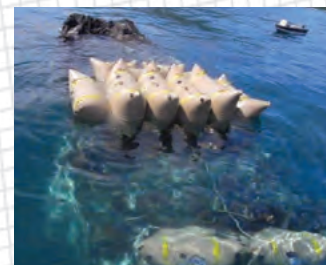
Shallow water wreck removal using clusters of Enclosed Flotation Bags 2,000 lbs.
