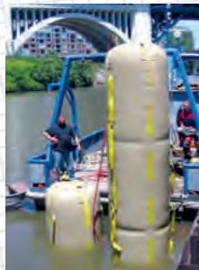
Custom Vertical Pontoons manufactured to allow accurate horizontal control during large pipe and valve maintenance and assembly.
