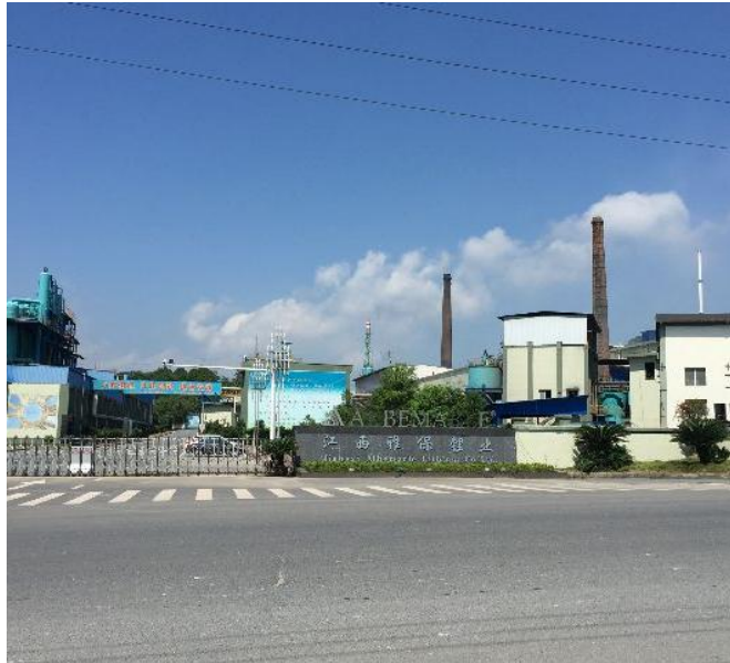
Albemarle Jiangxi 50,000 tons/year Lithium Hydroxide Project
