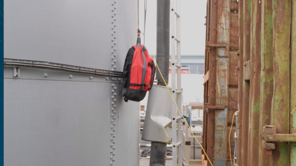
Fig2 Lift up the drone on the outside with a rope
