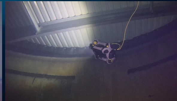
Fig6 Inspect high-level fittings on the tank
