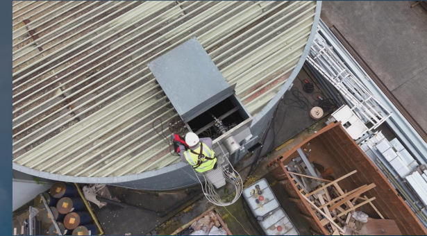
Fig3 Ready to enter the water tank
