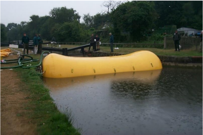
Flood Defence & Revetments
